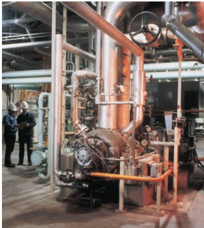
Feedwater pump. Photograph courtesy of Flowserve Corporation.
