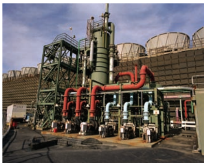
Condensers and cooling towers at The Geysers power plant in California. Photograph courtesy of NREL.
