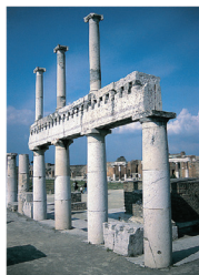
Part of the colonnade, which had two stories, seen from inside. You can see the holes for the floor beams of the top story.
