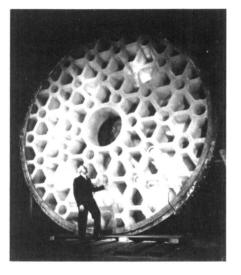
George McCauley of the Corning Glass Works with the completed 200-inch Pyrex blank for the ''Hale telescope.'' McCauley worked on a different design for the mirror's back, making it ribbed and leaving empty cells to improve the glass's response to changing temperatures. Photo courtesy of the Dept. of Archives and Records Management, Corning Glass Works.
