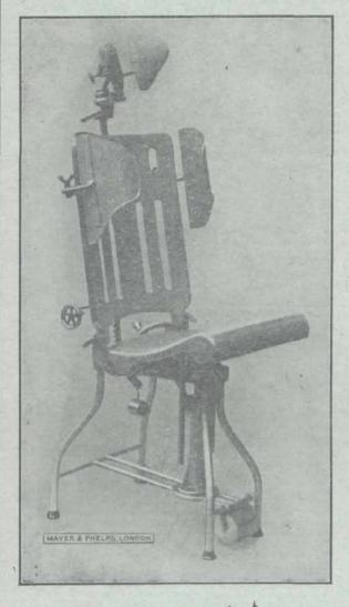
The Chair is designed for operative work on the head and neck under an anæsthetic and for general use in nose and throat work. It is sufficiently rigid for operations on the brain, mastoid, and gasserian ganglion.
