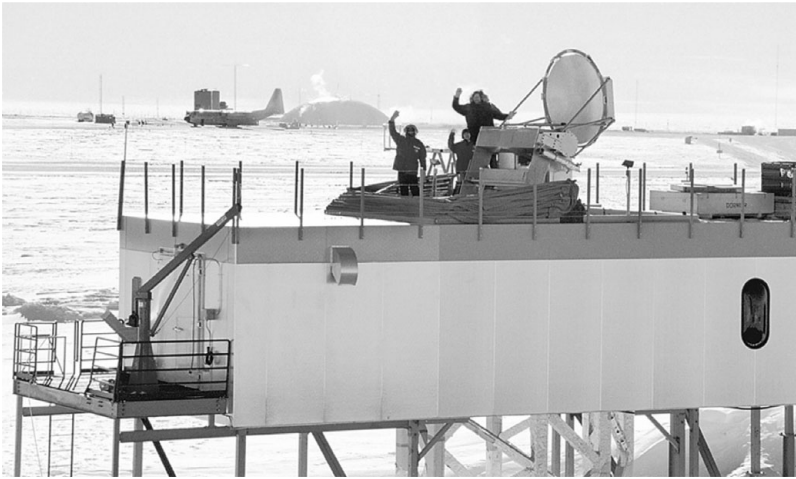
Figure 1. The AST/RO telescope and building. An insulated steel tower supports the telescope and extends through the building, which houses receivers and electronics in a shirt-sleeve environment. Photo credit A. Lane.
