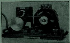
Rotary Blower with Electric Motor.
