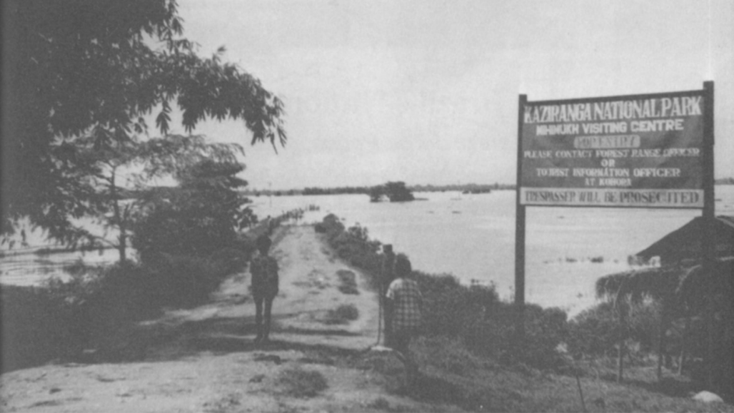
FLOOD WATER INVADES THE VISITING CENTRE, August 1973
