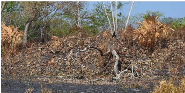
Figure 5. Photograph of Structure 12, illustrating the rubble fill spilling out of a platform that had its cut veneer stones removed. (Color online)
