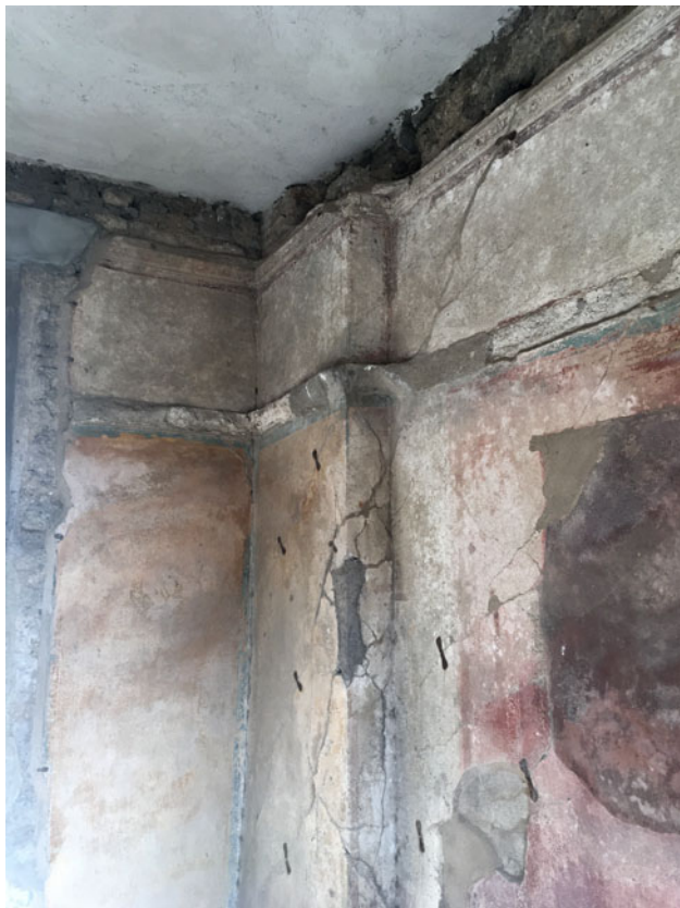
Fig. 7. Pompeii 9.2.5, south wall of "triclinium" showing projecting wall framing Pero and Micon fresco (removed). (K. Milnor. By Permission of the Italian Ministry for Cultural Heritage and Environment. Reproduction prohibited.)
