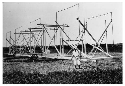
Figure 1.5 Karl Jansky and his Bruce Array at Holmdel, NJ, used for the first detection of cosmic radio emission. Credit: Nokia Corporation and AT&T Archives.
