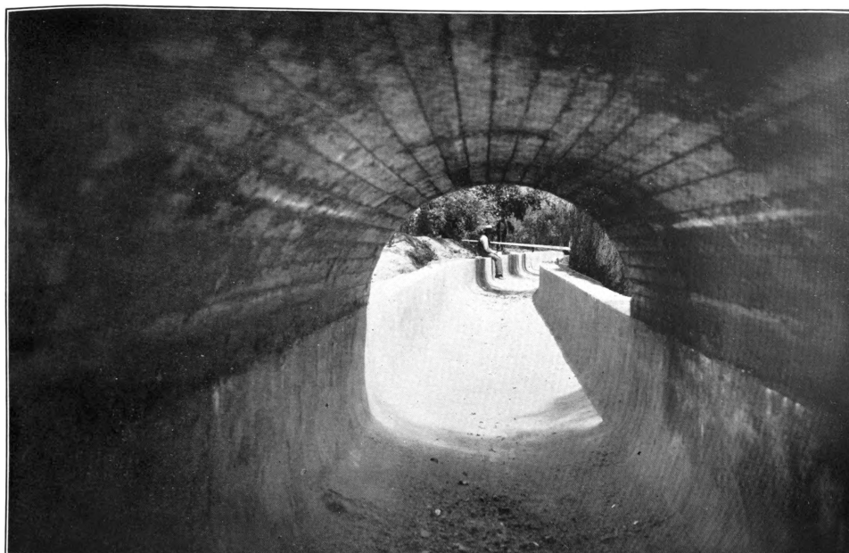
MAIN SUPPLY CONDUIT UNDER CONSTRUCTION
