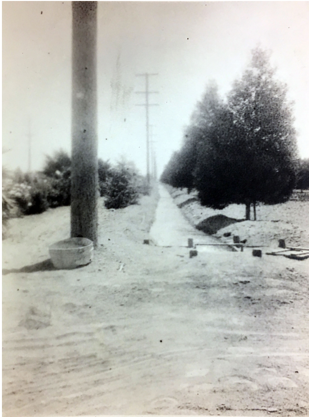
Figure 4. Lateral No. 1, three miles long, looking east along Sherman Way, San Fernando Valley, photo by C. F. Outland, c. 1915–1917. Historical Society of Southern California Collection, Huntington Library.
