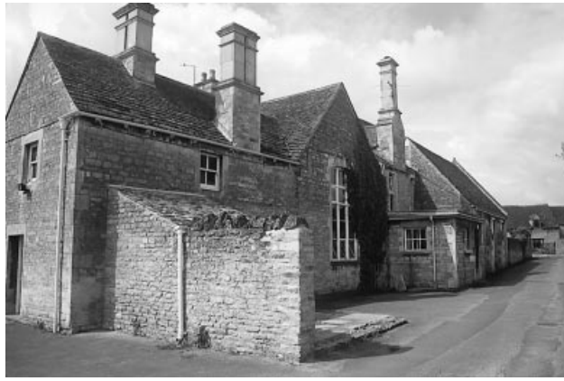
Fig. 4. Berkeley's house, King's Cliffe.
