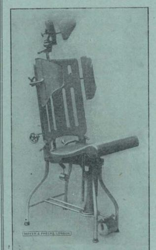
The Chair is designed for operative work on the head and neck under an anæsthetic and for general use in nose and throat work. It is sufficiently rigid for operations on the brain, mastoid, and gasserian ganglion.
