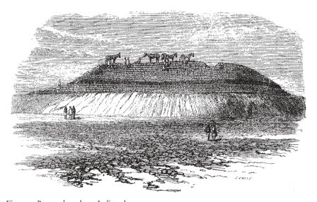
Figure 3. Puzawah, or large Indian clamp. Proby T. Cautley, Report on the Ganges Canal Works: From Their Commencement until the Opening of the Canal in 1854, 3 vols and one atlas (London, 1860), vol. 2, p. 197.
