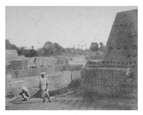
Figure 2. Clamps along the Hooghly river, near Calcutta, ready to be dismantled (right and left), with, in the foreground, stacks of green bricks drying, on which two workers are standing. Hand-coloured photographic print by Frederick Fiebig (c.1851–1852).
