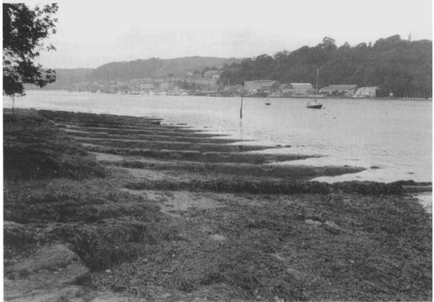
FIGURE 1. Gridirons at Lower Noss on the River Dart, Devon, photographed at low tide. (Photo J. Schofield.)
