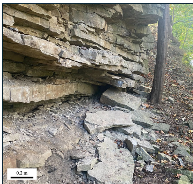
Figure 3. North-facing dolostone outcrop of the Gasport Formation at the Bruce Trail site (Site B) (43°14'38.9"N 79°53'12.3"W) showing recent loss of material through rockfall.
