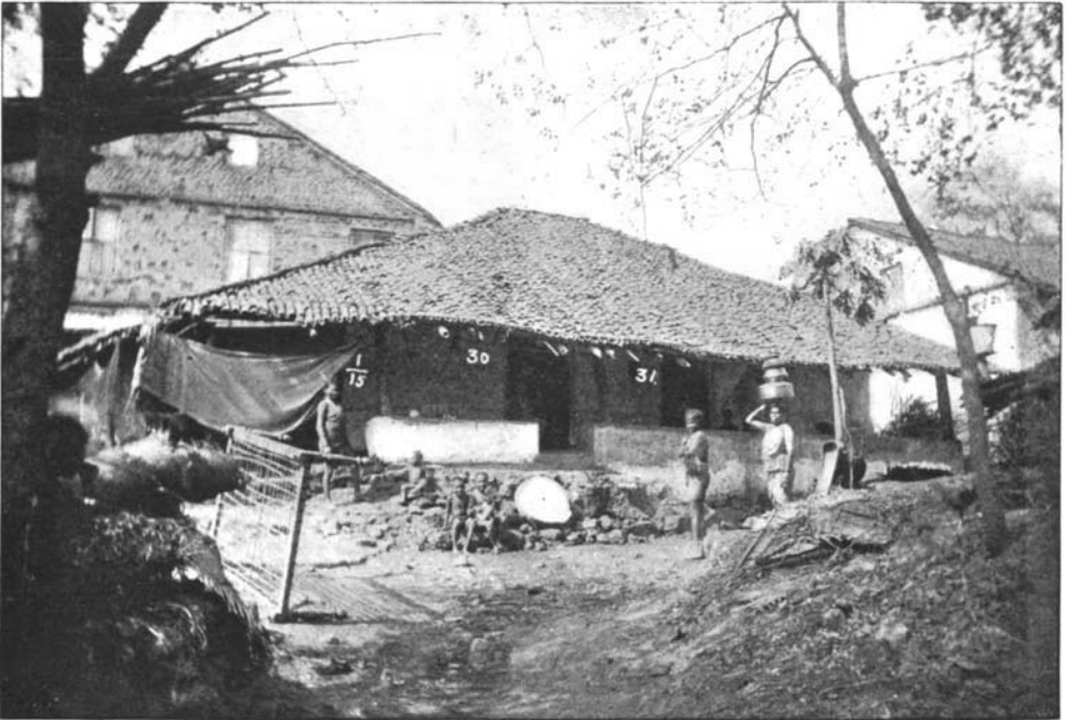
Sion Koliwada: showing tiles, verandah, etc.
