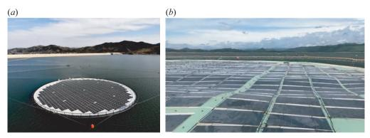
Figure 1. Floating solar: (a) 0.5 MWp floating PV system made by Ocean Sun, owned by Statkraft on their 72 MWp hydro power dam at Banja, Albania (Photo: Ocean Sun); (b) 0.22 MWp floating PV system made by Ocean Sun, owned by SNAP (SN–Aboitiz Power) located at the Magat hydro power reservoir at Isabela, Philippines (Photo: Ocean Sun).
