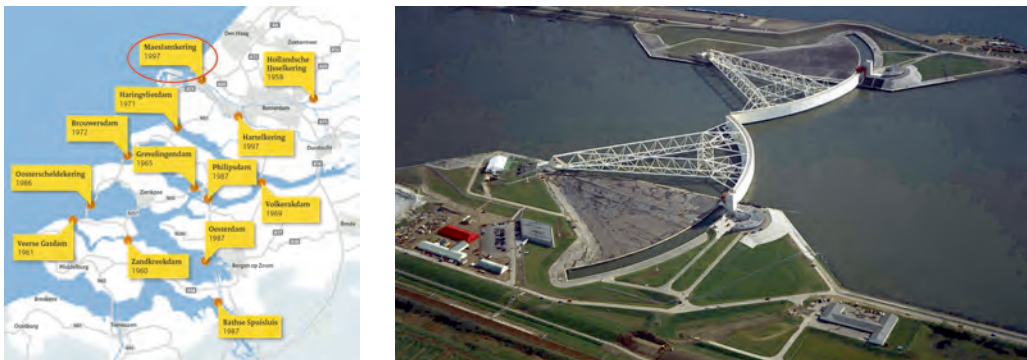
Figure 1.5 Left: The original 13 storm dikes and barriers from the Delta Works. Right: The Maeslantkering when closed. Sources: © Rijkswaterstaat (left) and Watersnoodmuseum (right)
