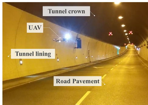
Figure 6. UAV inspection area as part of VCP 16 section in DPT.
