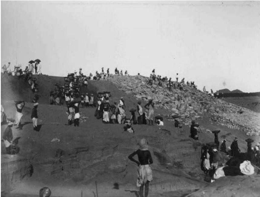
Figure 2. Kistna Bridge, Construction of the Western River-Training Embankment, c.1892. From an album "Kistna Bridge, Bezwada 12 spans of 30 Feet", F.J.E. Spring, L.C.E., M.I.C.E., engineer-in-chief. Held in the Library of the Institution of Civil Engineers, London and reproduced with the kind permission of the Institution.
