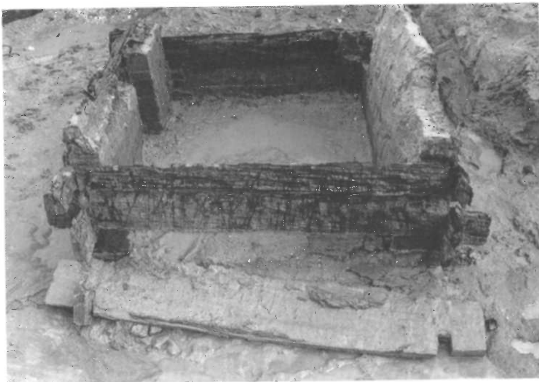
Fig. 5. Early Iron Age well (no. 1) of oak planks
