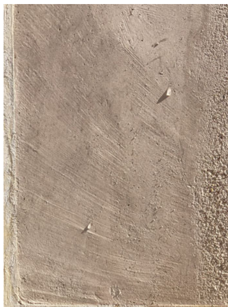
Figure 8. Polished opus signinum surface repelling water droplets. Note the trowel marks left in the process and the rougher, washed off surface, showing the difference between original finish and ‘archaeological’ state.
