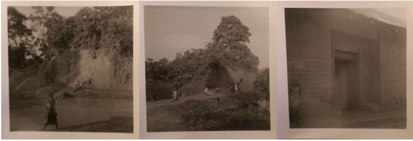
Figure 6. Photographs of Benin City architecture, including the inner earthwork, probably at Sakpoba Road where he excavated (left, centre) and the palace (right). The palace doorway shown here may be the one marked on his sketch map (above).
