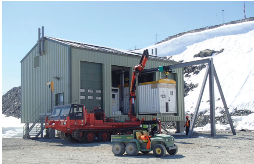
Fig. 4. The unique, purpose built A-frame gantry system for lifting and moving the units. Photo: T. Biggs
