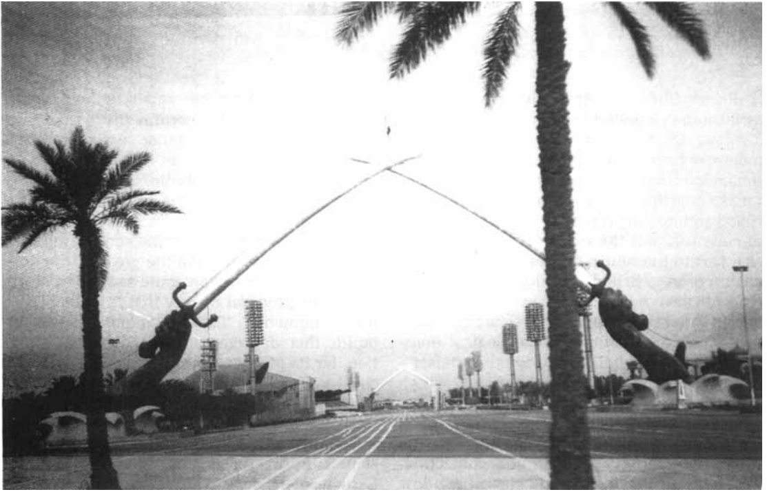
Saddam Hussein's monument, the twin Victory Arches in Baghdad, viewed along its ceremonial axis. Designed by Khalid al-Rahal and Mohammed Ghani, inaugurated August 1989. The swords, in cast steel, are some 40 m long, the arms and hands that hold them, in cast bronze, are some 16 m long.
