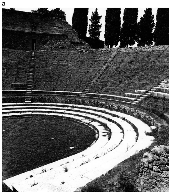
Figure 17a Large Theatre, Pompeii, showing subsellia (foreground), the cavea , the crypta and the area for seating at the top of the theatre, the summa cavea (top left). Photo: American Academy in Rome, Photographic Archive 11685.
