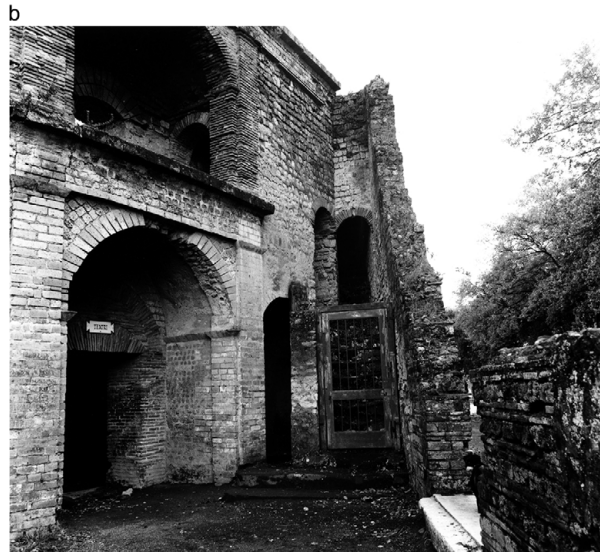
Figure 17b Entrance to the Large Theatre's crypta (left) and seating in the summa cavea (centre) from the Triangular Forum (right). Photo: American Academy in Rome, Photographic Archive 23702.
