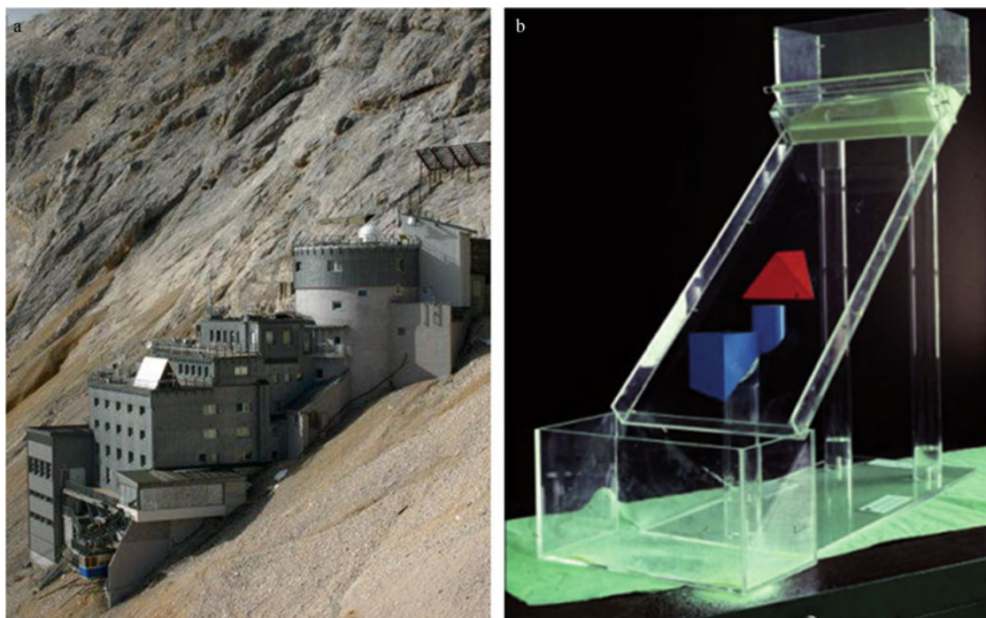
Fig. 14. (a) The Schneefernerhaus at the Zugspitze, Germany at 2700 m on a rather planar mountain slope inclined at \sim 45^\circ . (b) A model reproduction together with tetrahedral wedge type avalanche protection.
