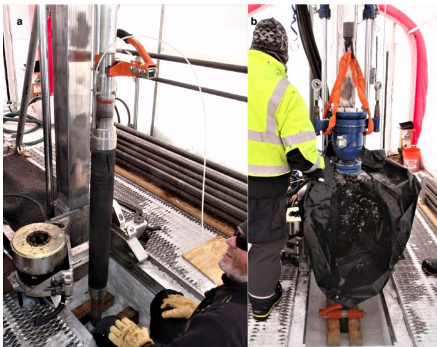
Fig. 4. (a) Inflatable packer installation. (b) Diverter and sump pit liner installation.
