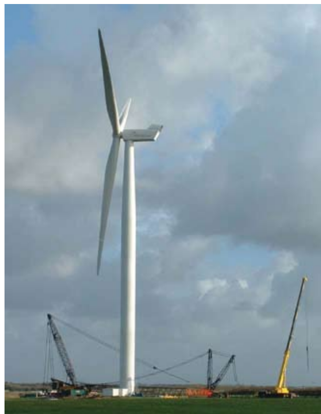
Figure 2. Modern wind turbine at Riso National Laboratory test site, Høvsøre, Denmark. The tower height is 120 m; the rotor diameter, 110 m; and the generator power, 3.6 MW.
