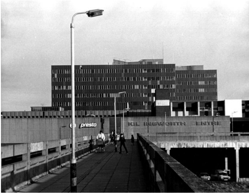
Figure 7—Places of “permanence and security,” part 2: The Killingworth Citadel “dominating the landscape” in 1983. In the foreground are the “low bastion” of the shopping mall and a “street in the sky” leading to the Towers. Deterioration is already evident in the missing sign letters, though the child on roller skates looks happy enough. Courtesy of Stephen Brain.
