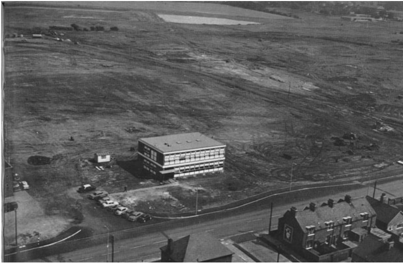
Figure 4—Developing the frontier: Killingworth Development Group offices, early 1960s. Courtesy of Northumberland County Council and Newcastle Libraries.
