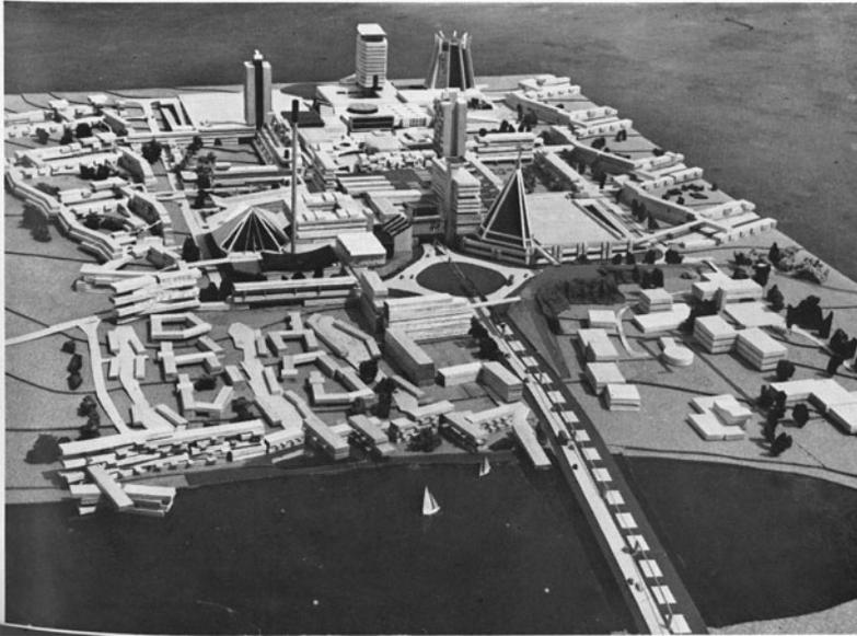
Figure 5—Model of Killingworth Township, facing north. The “walled town” effect was to be achieved through progressively higher building levels from the modest lakeshore housing on the fringe to the skyscrapers of the Citadel in the center. Courtesy of Northumberland County Council and Newcastle Libraries.
