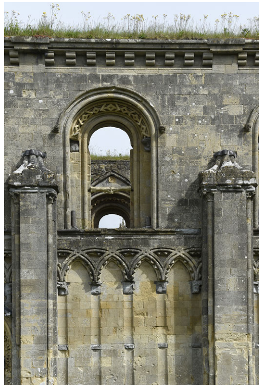
5.6 Photograph of Glastonbury Abbey’s Lady Chapel (Somerset) showing elements in the Romanesque style: round-headed windows with chevron decoration and intersecting blind arcading of round-headed arches with chevrons. Photograph by David Cousins © Glastonbury Abbey
