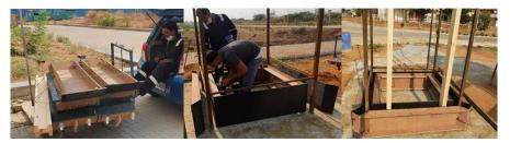
Figure 6: Transporting and installing the formwork at the site
