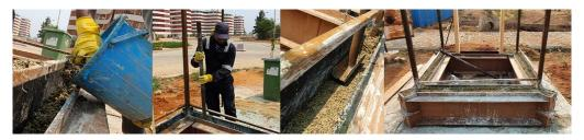
Figure 7: Pouring of Bio-Brick material, rand ramming and completion of the first layer
