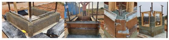
Figure 8: Photographs showing the layered casting of the wall
