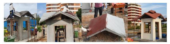
Figure 12: Finishing of the roof with cement plaster and cement punning
