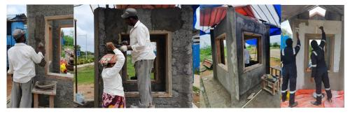
Figure 11: Plastering process of the Bio-Bricks wall
