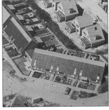
ON THE COVER: Ten family houses equipped with roof-integrated photovoltaic systems. Location: Heerhugowaard, 50 km north of Amsterdam. Each system is approximately 1.5 kW-peak and connected to the 220 V grid. Systems are operated by the PEN Utility Company of the province of North-Holland. (Photo kindly provided by PEN.) For more information on materials for photovoltaics, see the section beginning on page 18.
