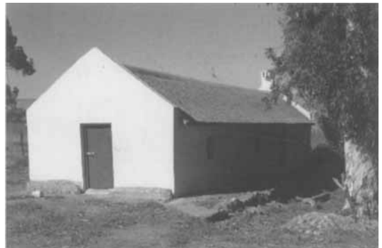
Elandsbaai: the University of Cape Town field station above the vlei is a langhuis. Thatch and whitewash keep its mudbrick sound, by the usual rule that mud buildings need a good hat, a good set of shoes, and a good coat to keep safely dry.
