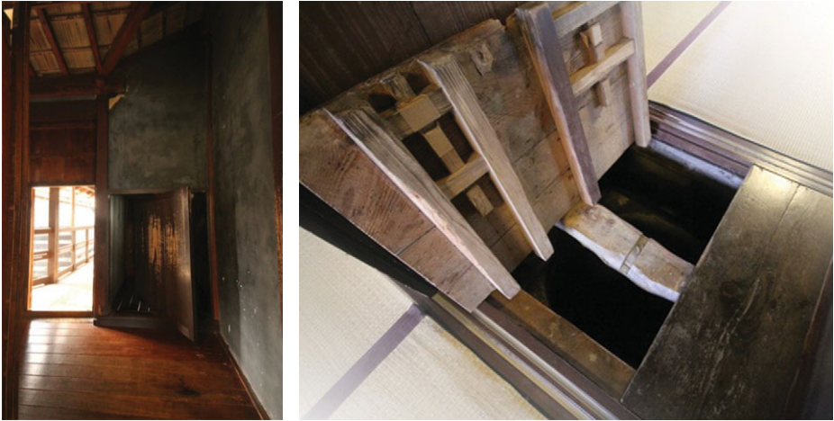
Figure 1.7 Pictures from the Kouka-ninja house in Kōka showing a revolving wall (left) and a trap (right) for hiding from possible enemies.
