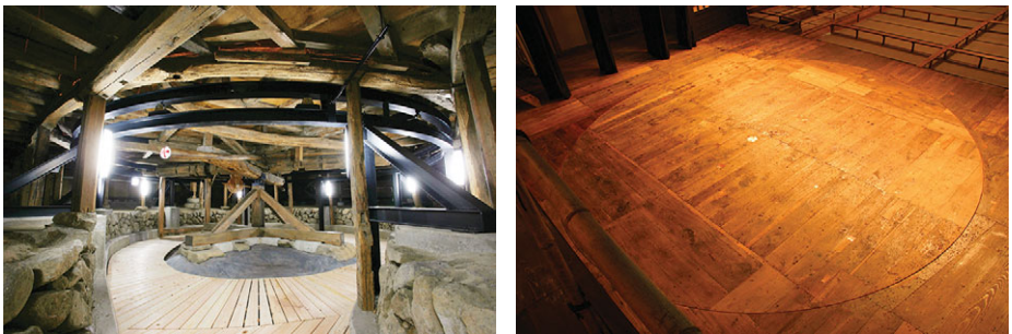
Figure 1.8 Revolving stage or Mawari-butai Karakuri. Images from Izushi Eraikukan[30]
