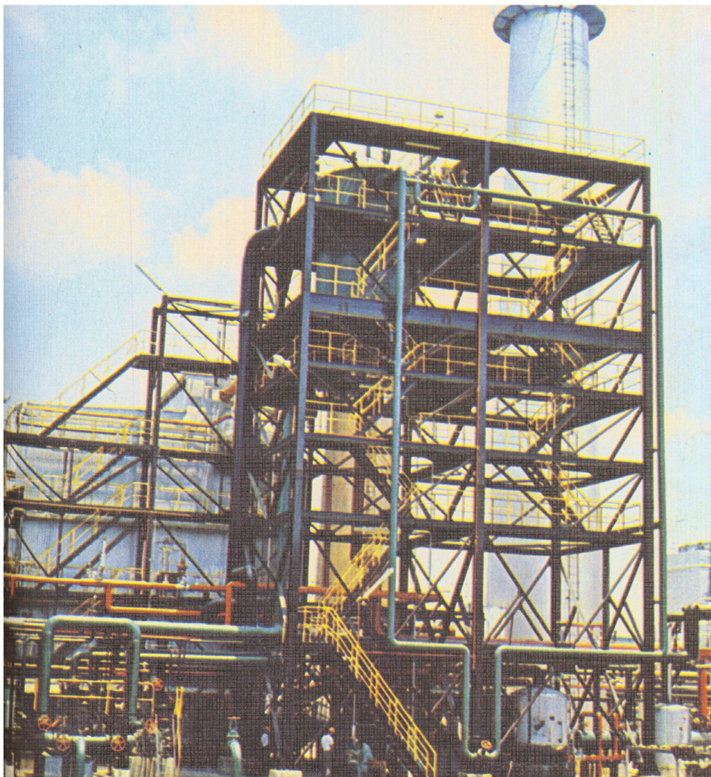
Figure 6. A large industrial boiler manufactured and installed by TMMC for Chinese Petroleum Corp. in Kaohsiung in 1971. This boiler has a capacity of producing steam at a rate of 240,000 lbs per hour. Taiji yuekan 8.5 (Oct, 1971), cover.
