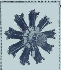
The Jupiter Engine is the lightest proved engine of its power in the world. It is the only aero engine which has passed both the British and French official tests. It has also completed an official test of 150 hours at 90% full power, including a 50 hours non-stop run.
