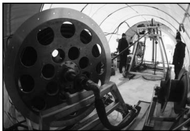
Fig. 2. Set-up of the AMISOR HWD drill tent with hose winch in left foreground and capstan stand over the borehole in right background.
