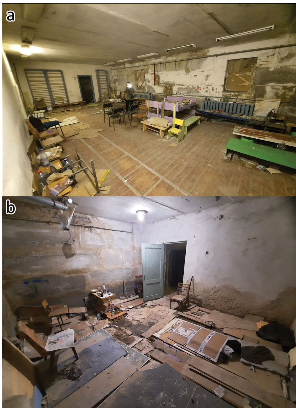
Figure 4. Interior of the school basement: a) the largest basement chamber, originally a gym; b) a room insulated with cardboard and ping-pong tables, 11 June 2023 (photograph by M. Lemiesz).
