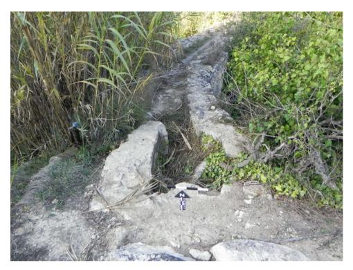
Fig. 7. Rock-cut tank at south end (i.e. the start) of the Agios Sozontas Bridge (with metal pipe embedded in bridging channel).
