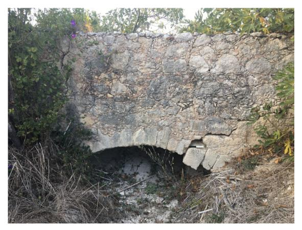
Fig. 12. Ampela Bridge 1, south face. Note crack and slipped voussoirs along right side.
