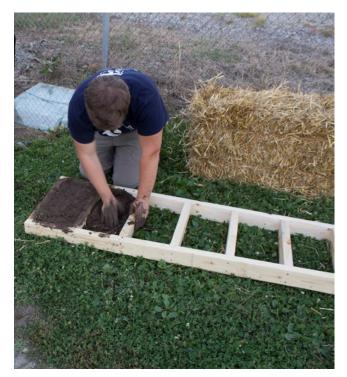
Figure 1. | Making mudbricks in a wooden mould.
