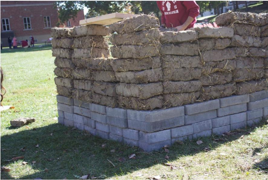
**Figure 4.** | The construction of the building's walls.
