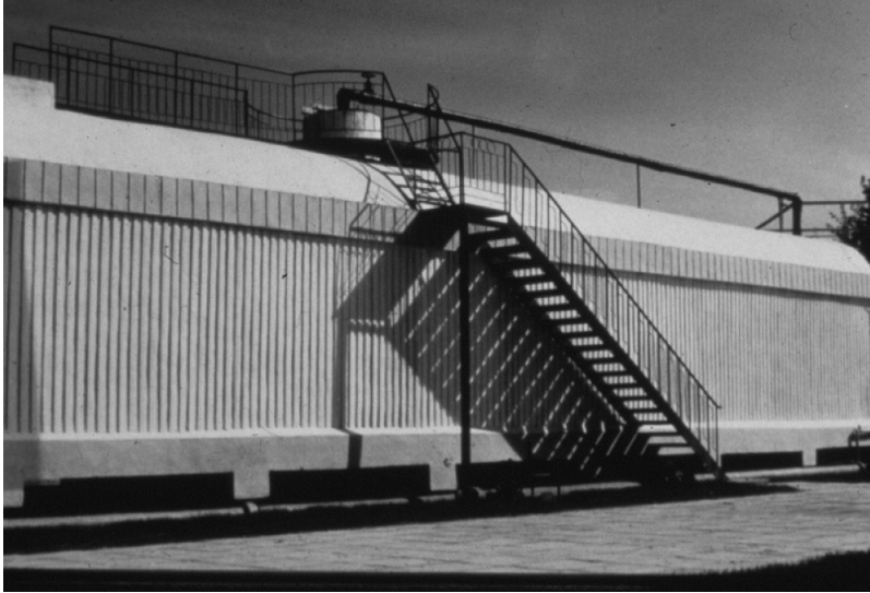
Figure 3 100-m 3 Liuminying digester for 50,000 hens in Beijing.
