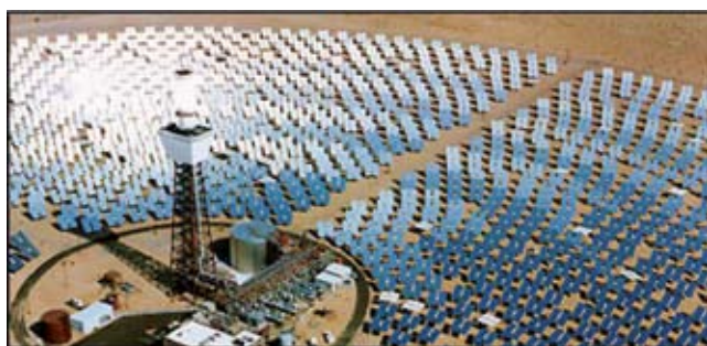
Figure 10. Solar 2 power tower in Barstow, California. The plant uses a combination of 60% sodium nitrate and 40% potassium nitrate as a working fluid and heat storage medium.
