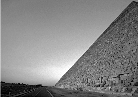
Fig. 160 The western baseline of the Great Pyramid. Beyond the narrow levelled strip of rock beside the baseline – half of which is now covered by the modern road – there is a considerable cut excavated by the pyramid-makers as they quarried out the platform for the Pyramid from the slope of the Plateau. By the tenth year of Khufu's reign, tombs were already being built upon the sloping hillside up above the Pyramid, as some of their building graffiti show (see further pp. 412ff below).
