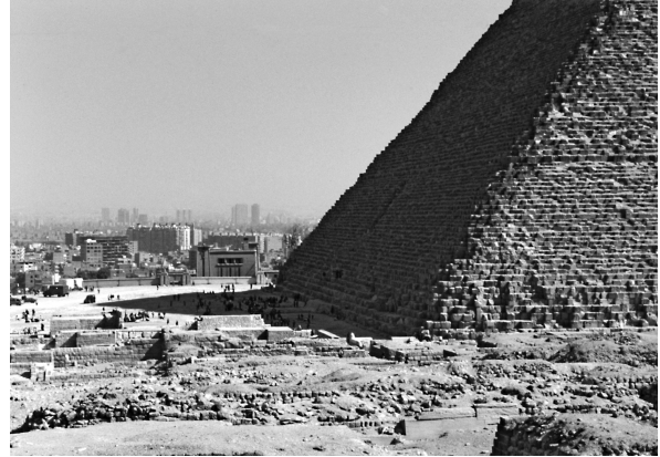
Fig. 161 The levelled area to the north of the Great Pyramid was yet narrower when building started on the Pyramid, before hundreds of tons of building debris were tipped down from the cliff top; the hard rock on which the Pyramid is set barely extends beyond the area covered by the shadow in this photograph.
