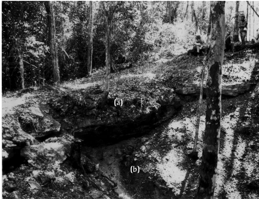
Figure 9. The side of a natural limestone causeway sloping down from the inner edge of the ditch (right). (a) The hard caprock is being undermined by (b) erosion of the underlying softer sascab . Photograph by the authors.
