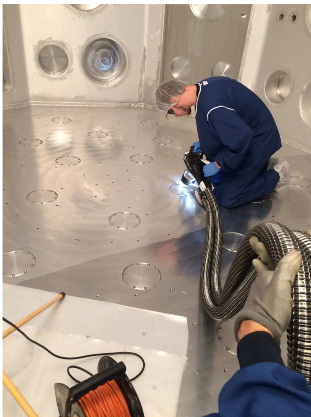
Figure 19. Cleaning of the P3 chamber floor shows a clear visual difference between the cleaned surface area and the non-cleaned area [31] .
